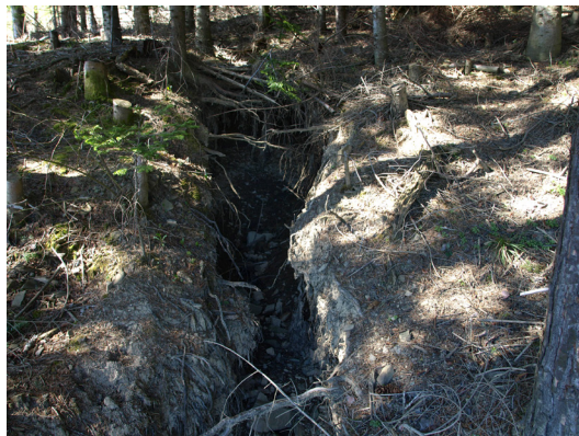
Fig. 3. Erosion ravine, depth of 1.5 m formed by accumulation of surface water runoff from several forest roads in the village of Slovenská Ves (April 20, 2011, photo: J. Slivinský)
