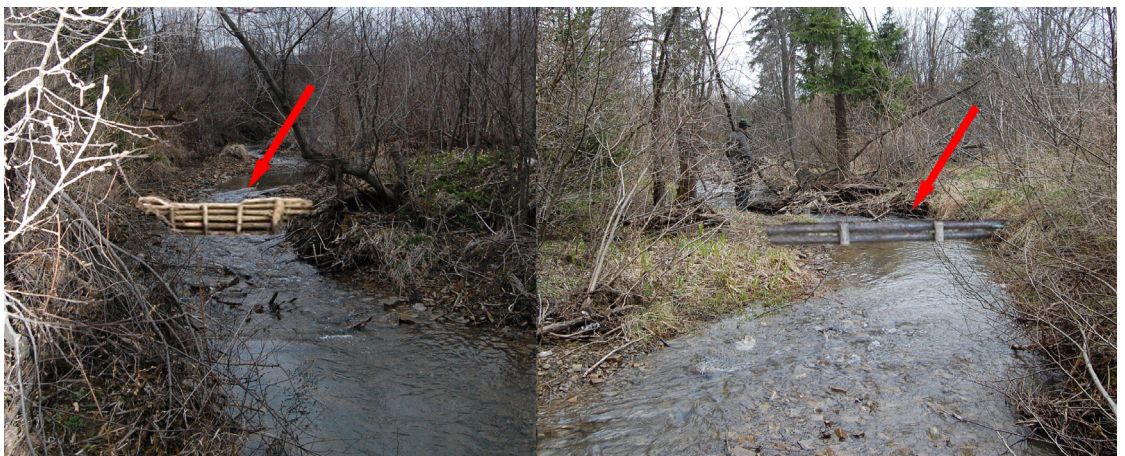
Fig. 9. Slovak creek (17 dikes) – sills, steps, dikes (April 15, 2011, photo: M. Janiga, simulation of waterholding measures)
