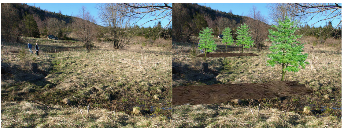
Fig. 10. The absorption ditch with retention area (left – present state April 20, 2011, photo: J. Slivinský, right - suggestion flood measures)
