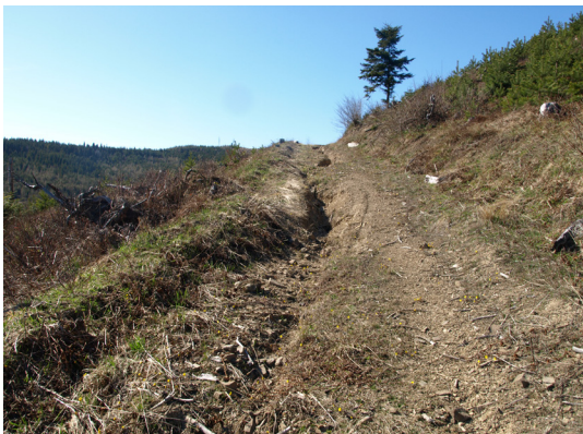
Fig. 2. Erosion groove caused by runoff (April 20, 2011, photo: J. Slivinský)
