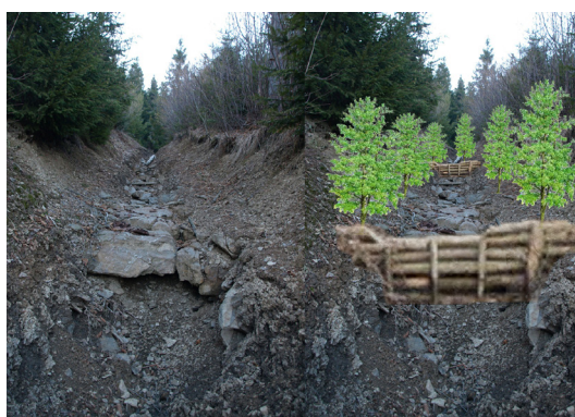
Fig. 7. The proposed model of water dikes in forest erosion groove (left - the current state; April 20, 2011, photo: J. Slivinský, right - suggestion flood measures)
