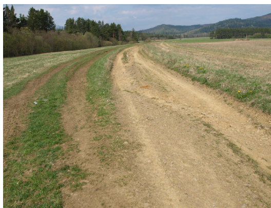
Fig. 5. New parallel field road along original field road in the village Slovenská Ves (April 20, 2011, photo: J. Slivinský)
